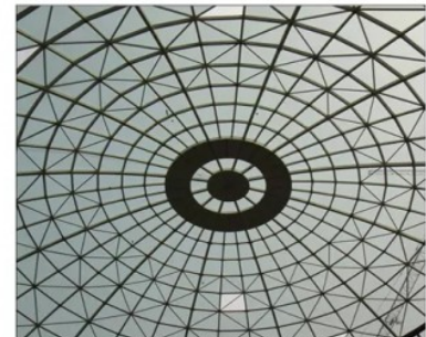
Suit for sunlight room sealing and gap filling
